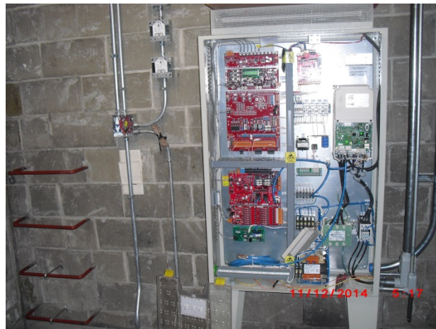
New Elevator Controls installed in the State House in December 2014. These electronic controls replaced the old relays and switches that were installed in the 1960's. The elevator now has fire recall and meets the current elevator codes.
